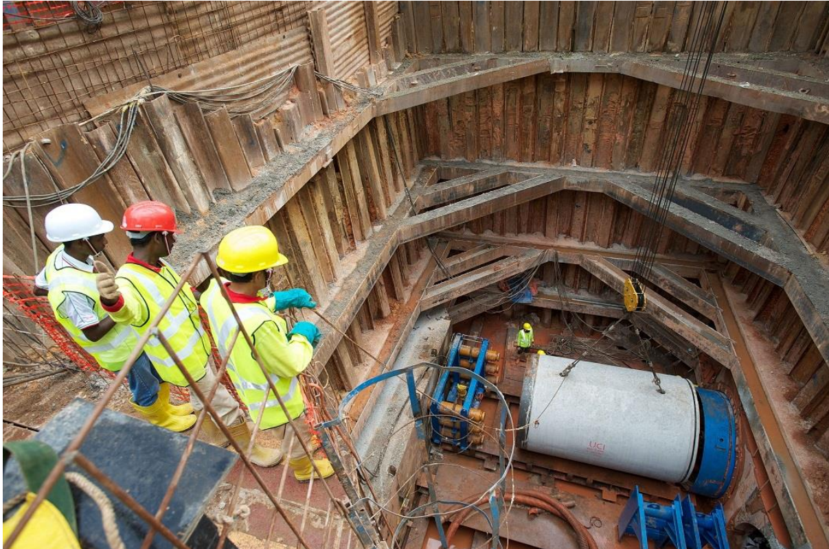
Ley Choon’s micro-tunnelling in action in a past project
