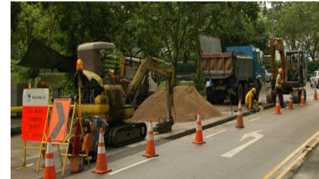
Road works in Singapore for cable laying
