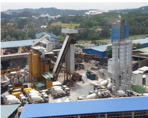
Operations in Ley Choon's neighboring plant, note the congestion of vehicles and lack of storage space.
