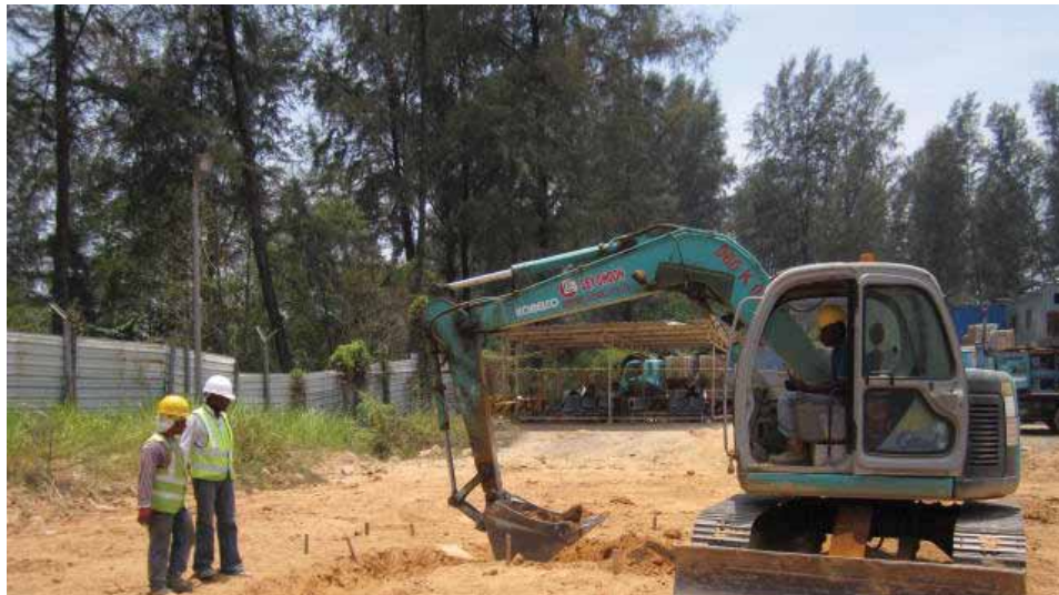
Training on Hydraulic Excavator operations
