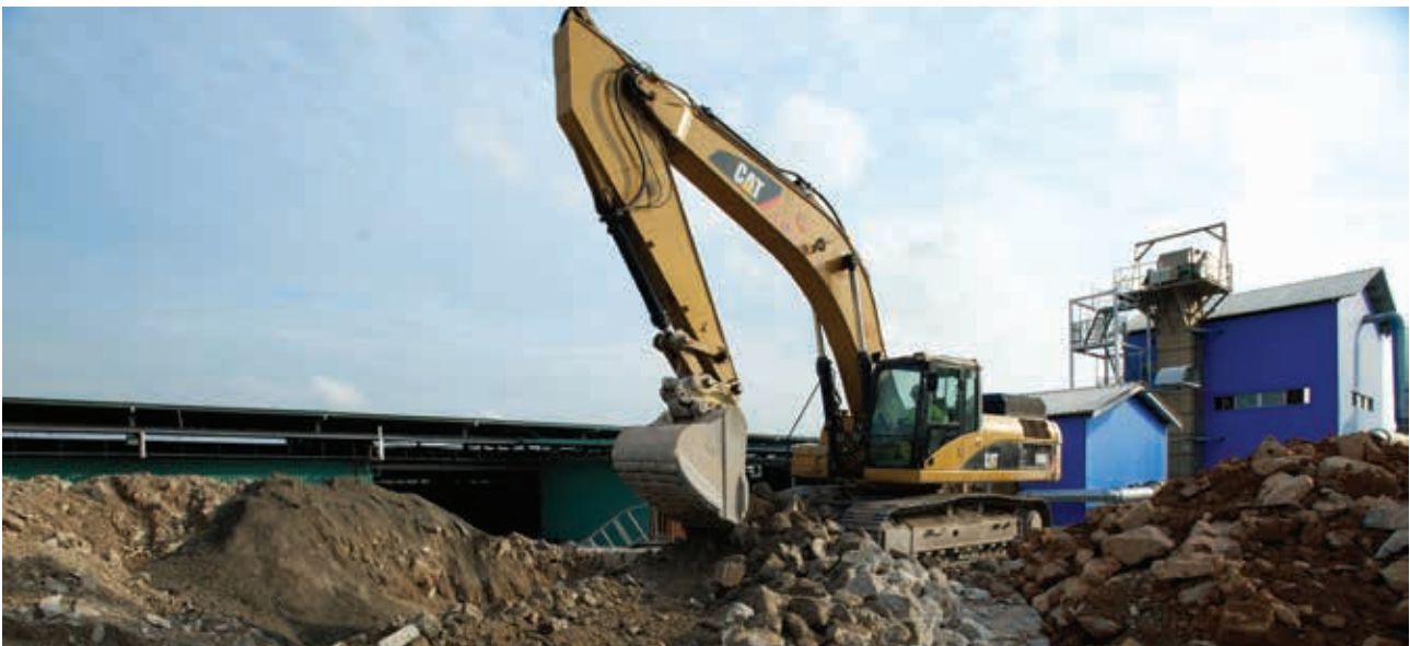
Construction waste recycling
